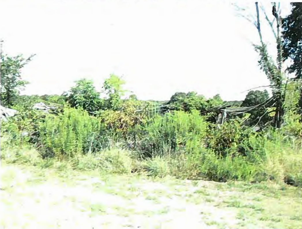
Date: 08/15/2012 Time: 10:05 a.m. Direction: north Photo by: Garrison Gross Exposure #: 010 Comments: collapsed building / demolition debris
